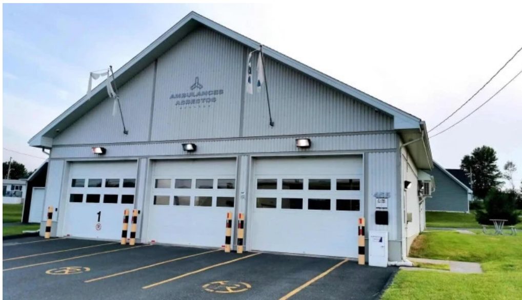
Dessercom asbestos all
