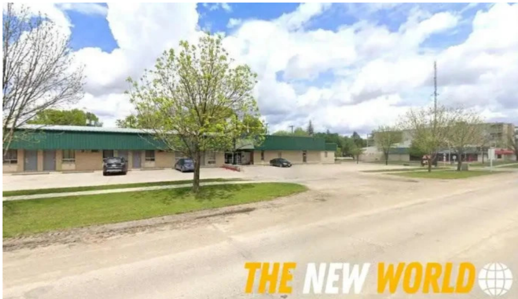
Centre point plaza altona
