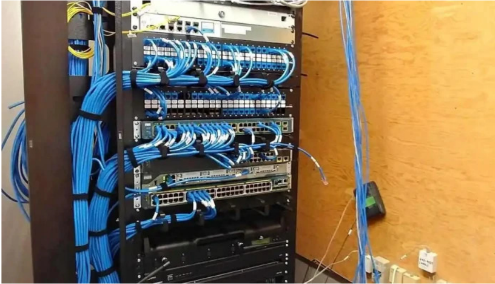
First response technical services inc by owner
