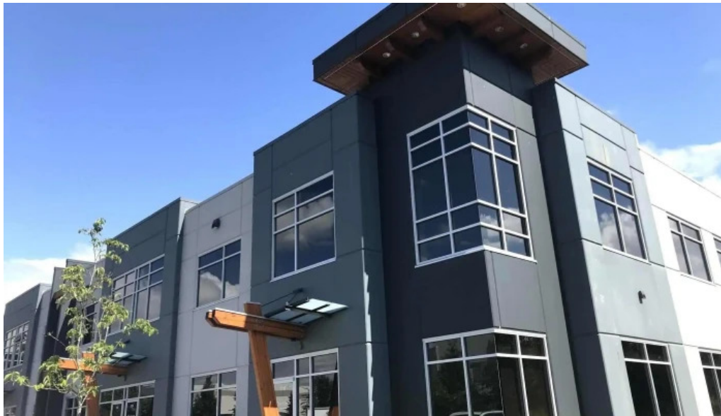
Activeco technology management by owner
