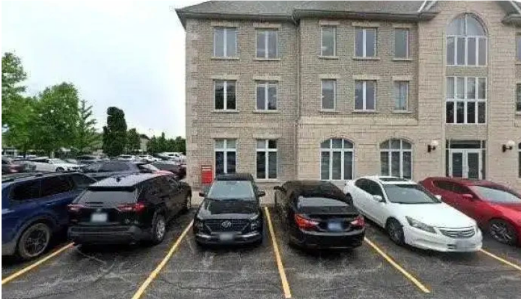
Robinson consultants inc all
