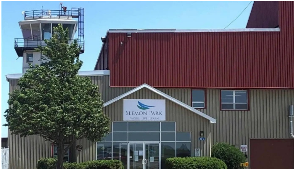
Dynamic controls canada inc by owner
