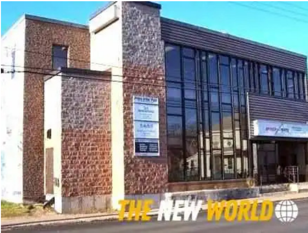
Amherst service canada centre building
