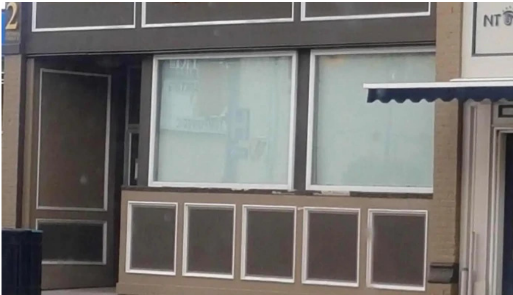
Feehely gastaldi barristers and solicitors alliston exterior
