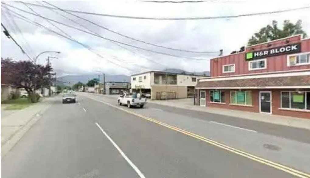
Combined workplace safety consulting street view 360
