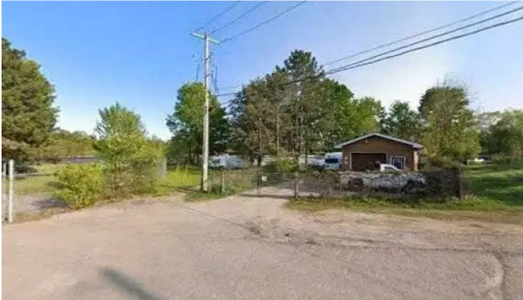
Arnprior sewage system upgrades all
