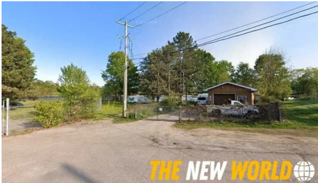
Arnprior sewage system upgrades arnprior
