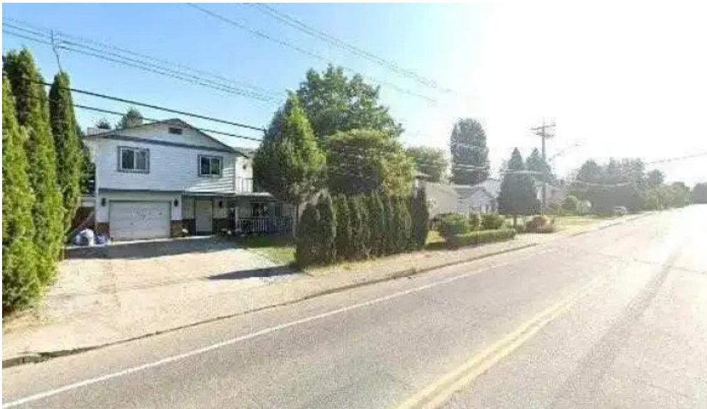
Safetecton inc street view 360deg
