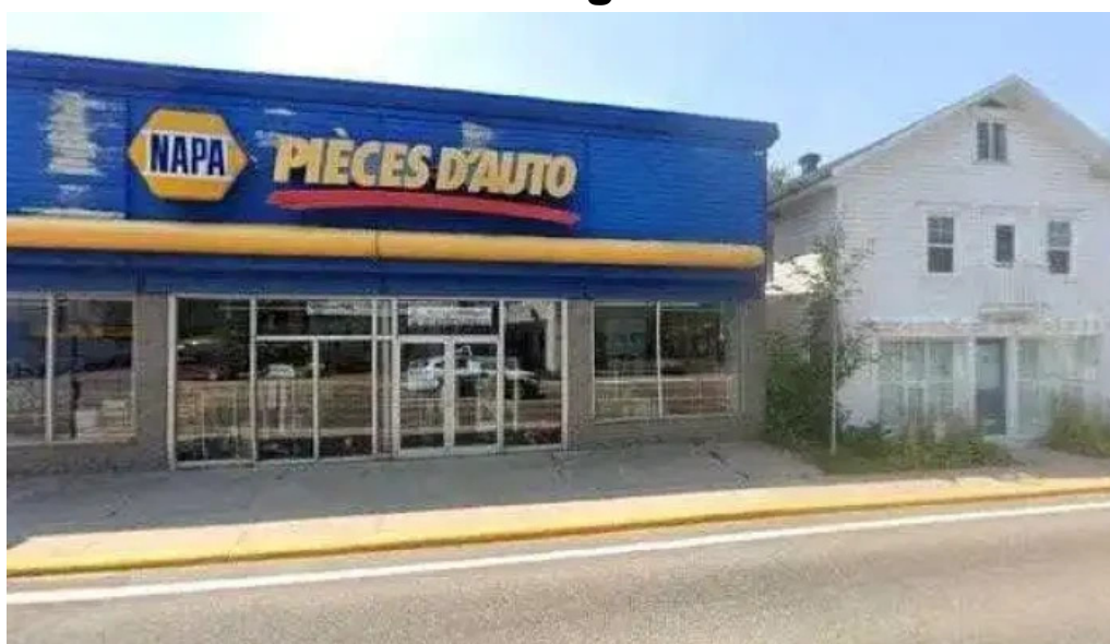
D modules street view 360deg
