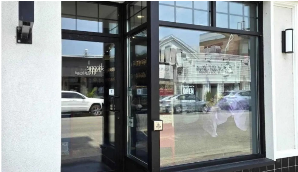
Atb solutions exterior
